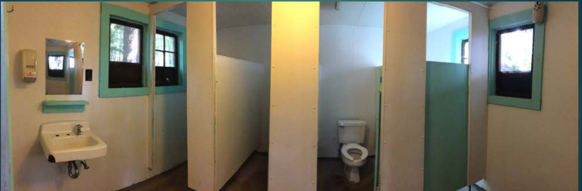
Comfort Station Interior
