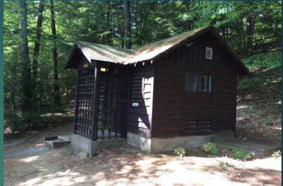
Beach Road Comfort Station (11)
