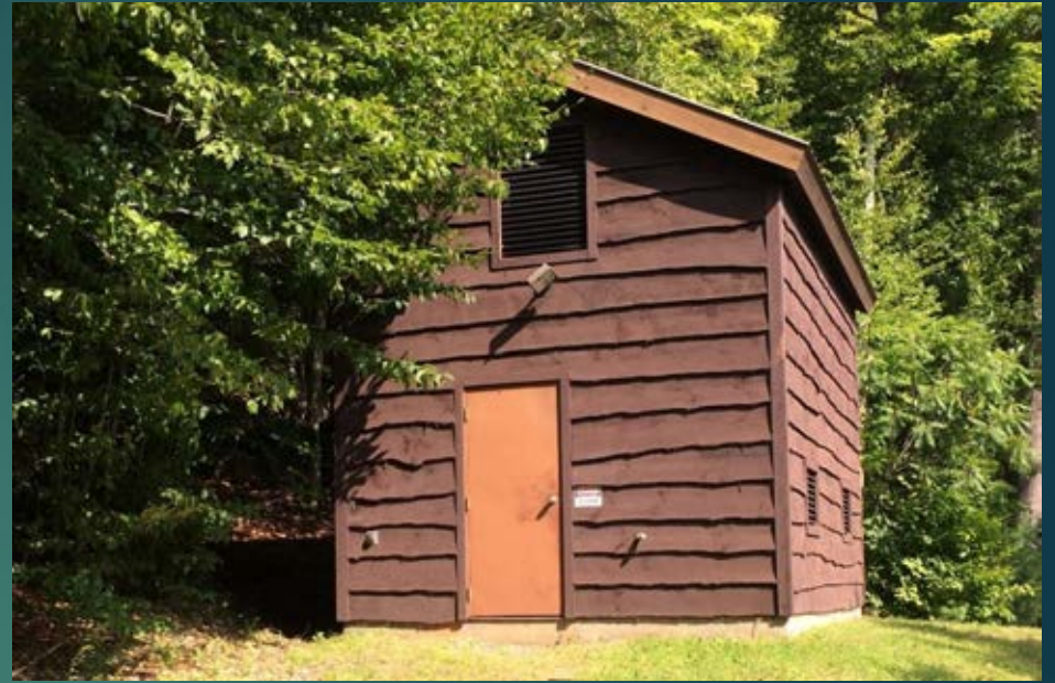
Chlorination & Reservoir Bldg
