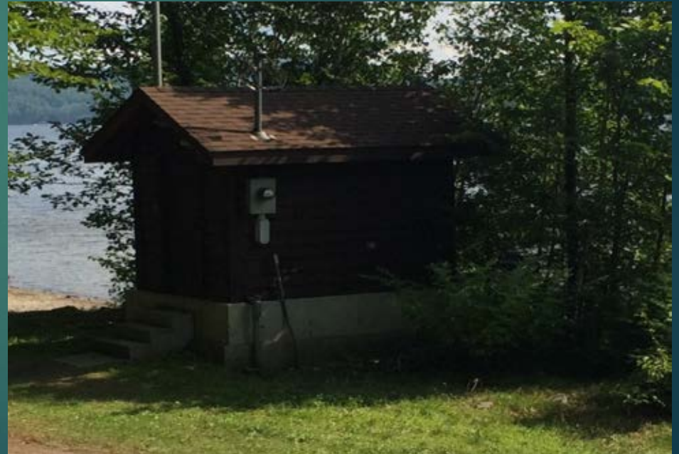
Water Pump House (16)
